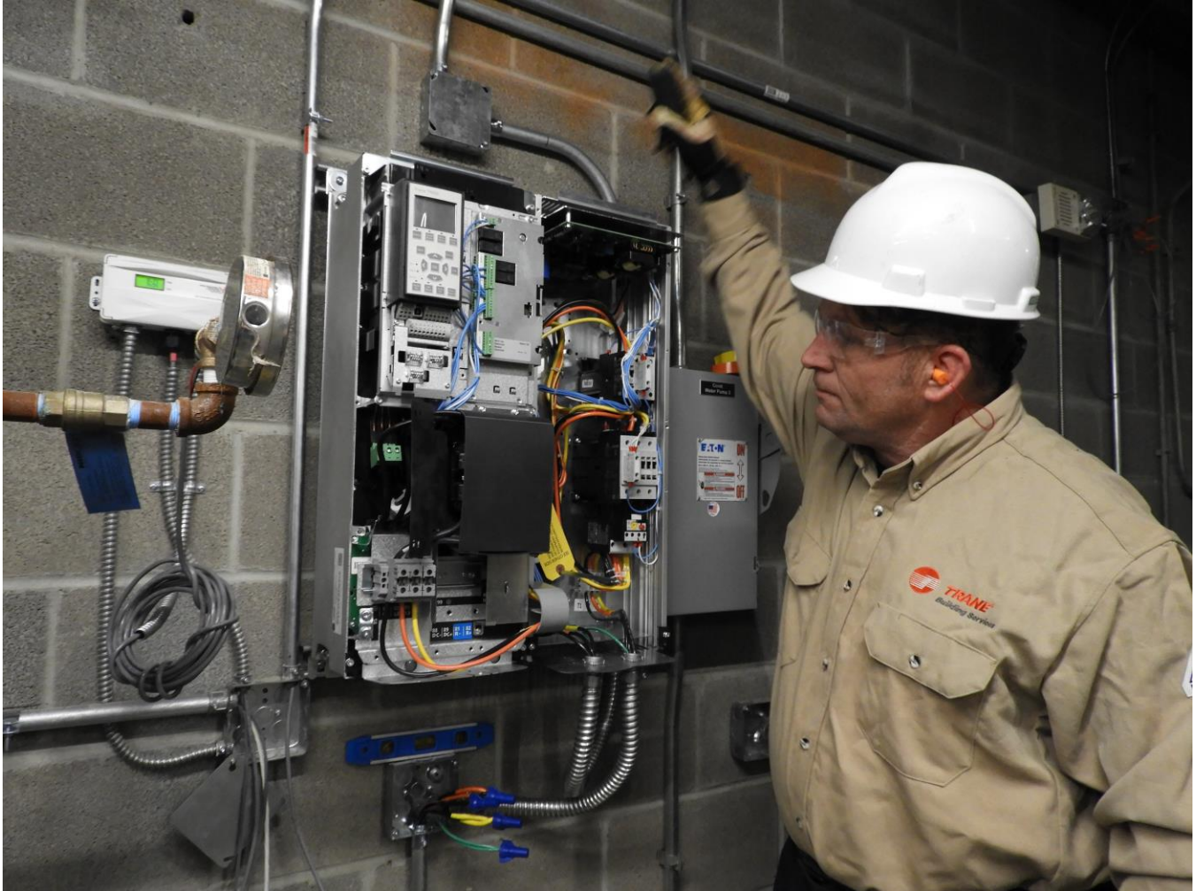
Custom Commercial project: Chiller/Controls/Variable Frequency Drive (VFD) upgrade project by registered trade ally, Trane.
