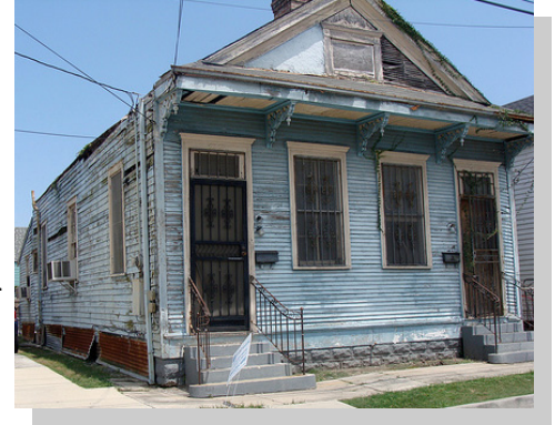
The home after Hurricane Katrina
