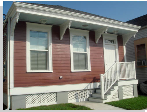
The rebuilt home on Soniat Street
